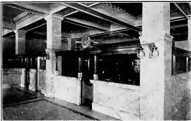
Interior View, Central National Bank
